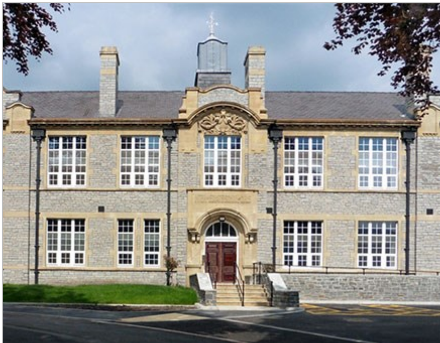
The former Aberdare Girls County School
