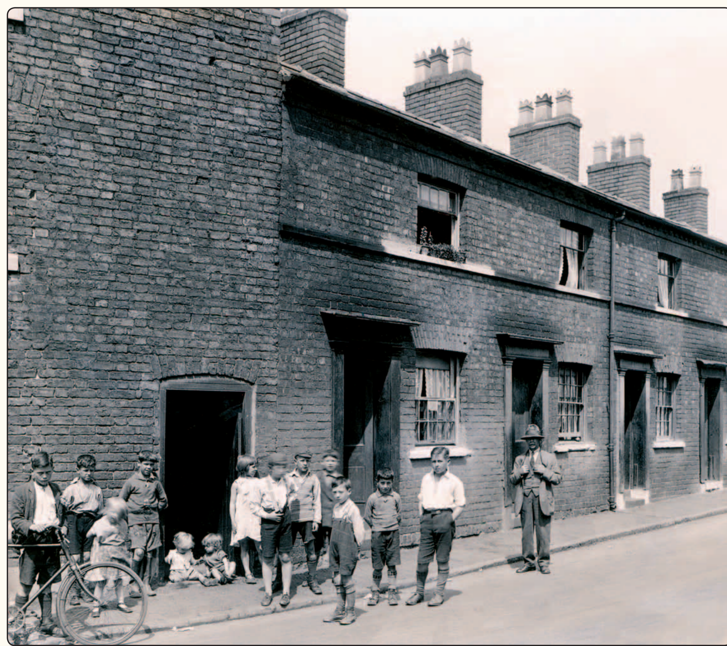
Condemned housing on Farndon Street. Tai a gondemniwyd ar Farndon Street.
