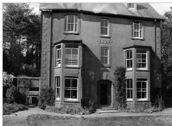
Neuadd-y-Wenallt, c1943. Between the first and second floors is the date 1897
