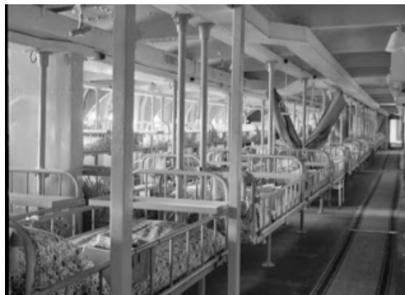
Typical cot arrangement in a Hospital Ship Ward
