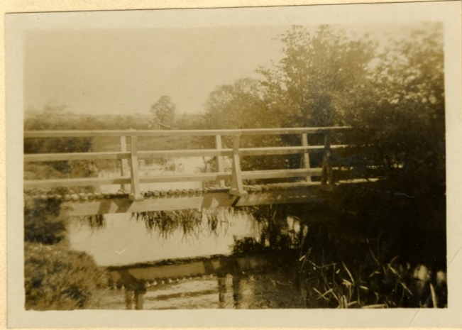
Wooden bridge crossing the Shaw.
