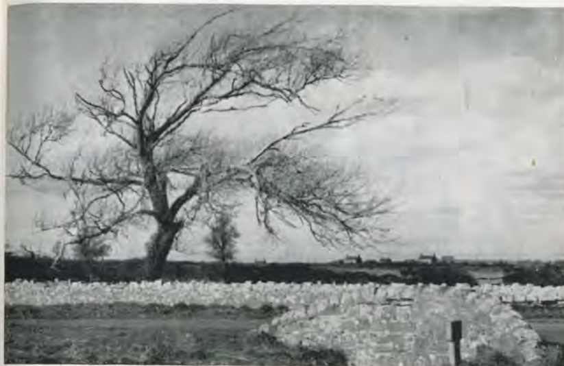
Fisher's Bridge, near St. Athan
