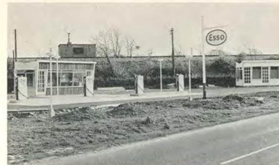
FOUR CROSS SERVICE STATION
