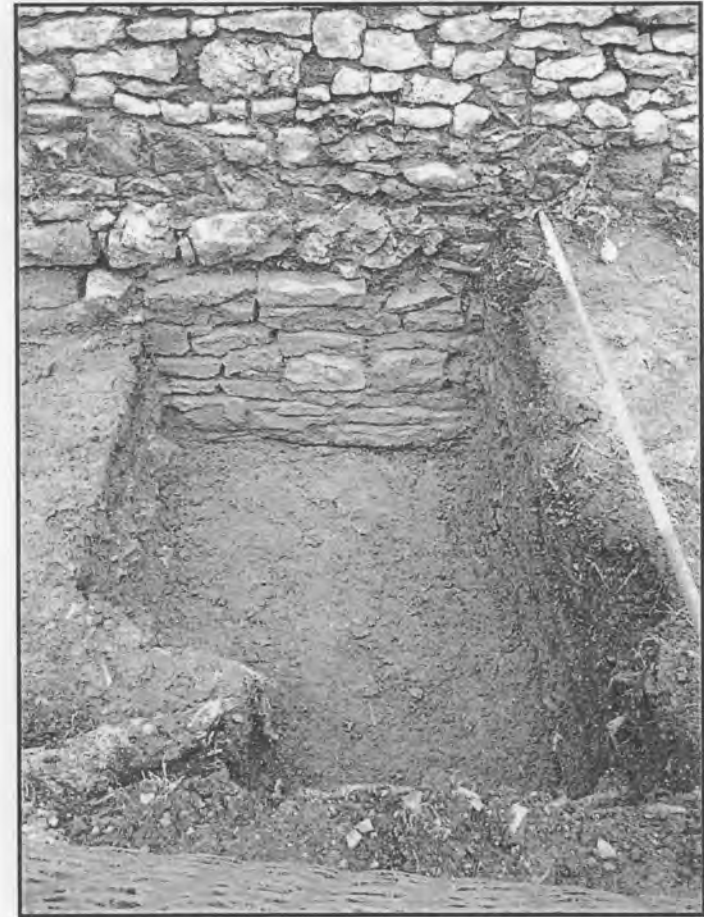
Plate 5: TP2, the medieval wall below the 18 th century wall from the north (CAC 2007, pl.16)
