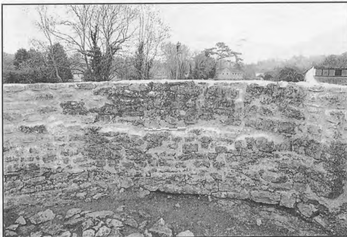
Plate 10: Repaired section in the eastern summer-house wall from the east
