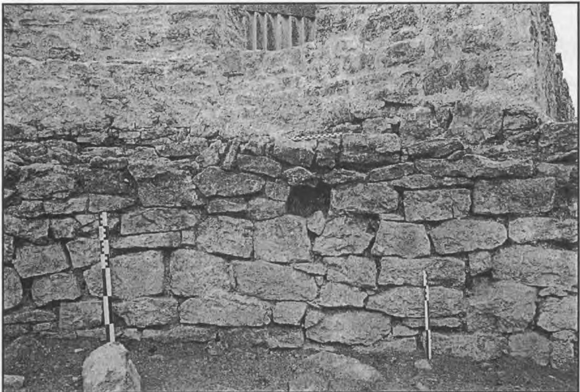
Plate 19: the northern revetment wall in the tower from the south
