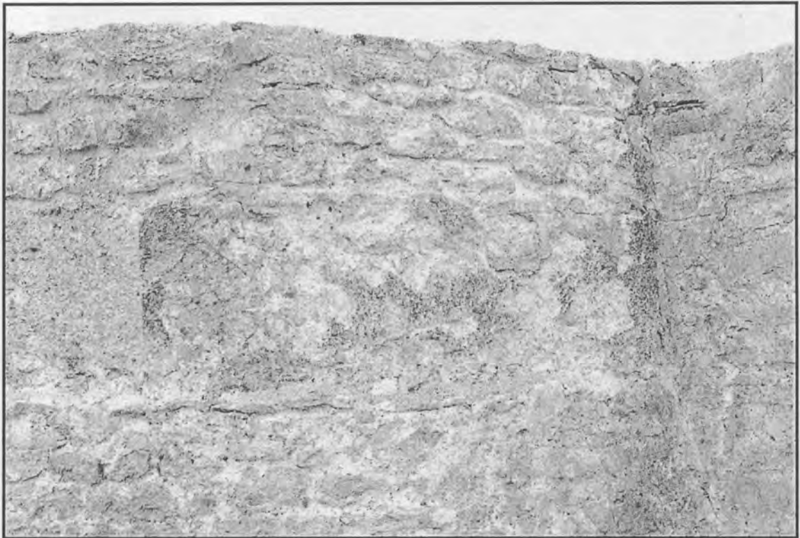
Plate 9: Remains of the gravel render on the external summer-house wall from the east
