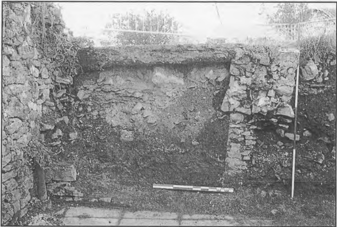
Plate 26: The retaining wall of the raised walkway from the north
