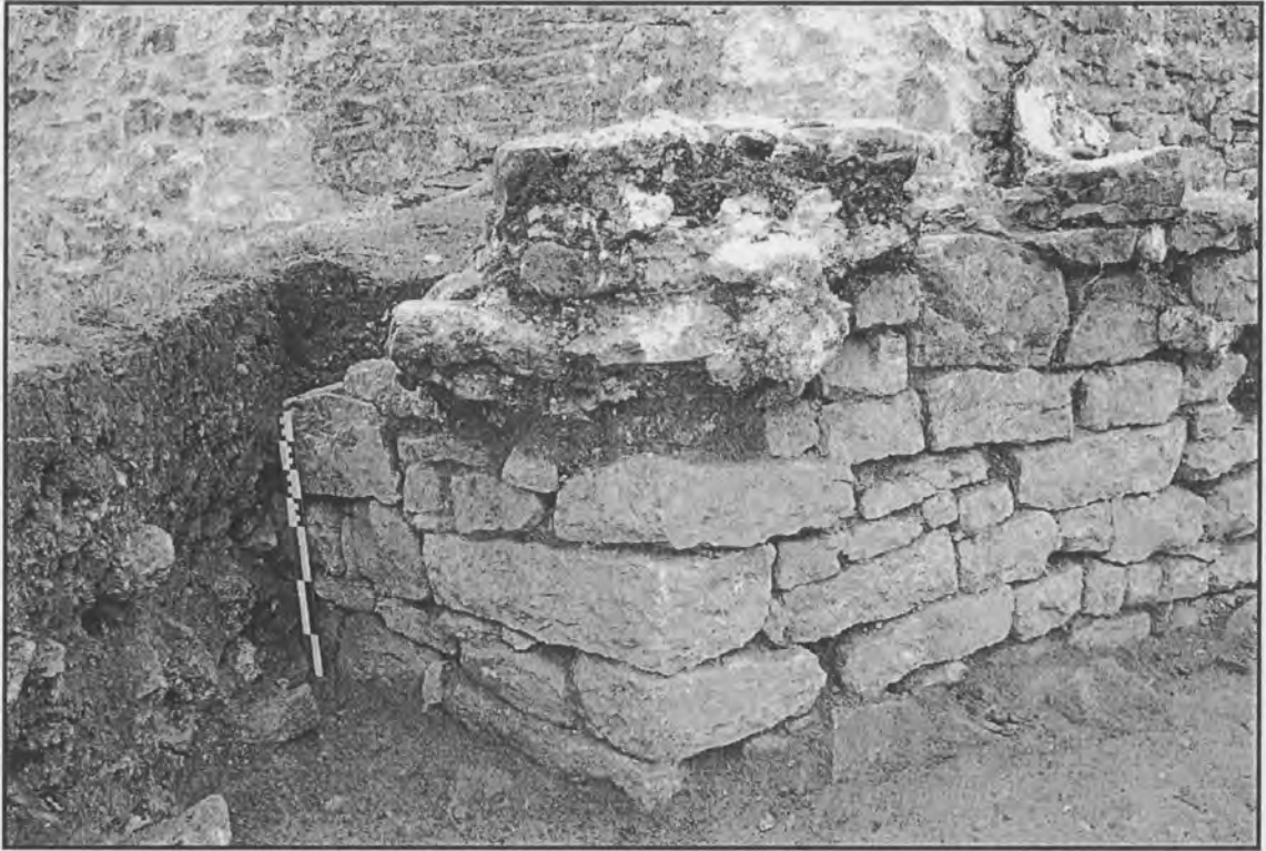
Plate 16: South-east corner of the tower from the north
