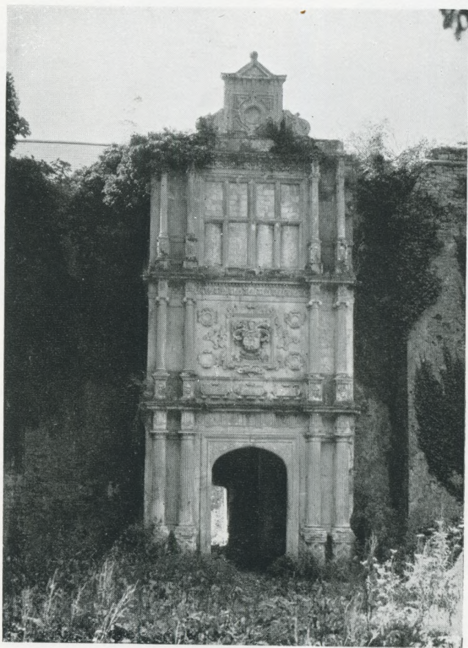
CASTLE OF OLD BEAUPRE—MAIN ENTRANCE PORCH—ST. HILARY Ernest Carver & Son Ltd., Bridgend
